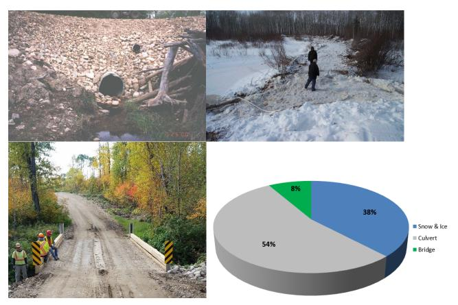
Figure 3-1: Examples of crossings - round culvert, snow and ice, portable steel bridge, and the percentages of each proposed crossing type.
