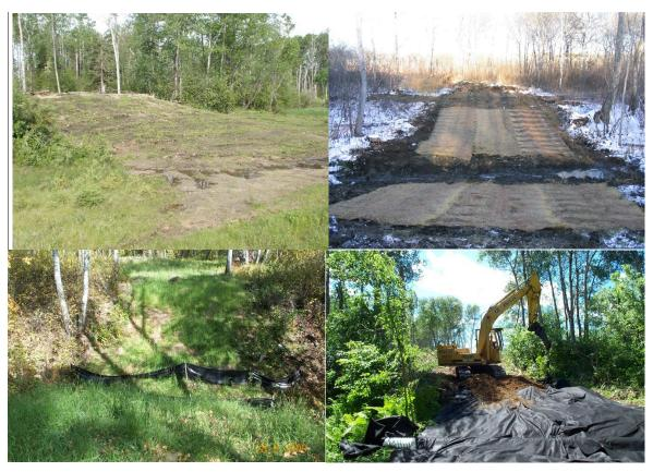
Figure 3-2: Examples of water crossing erosion control methods.
